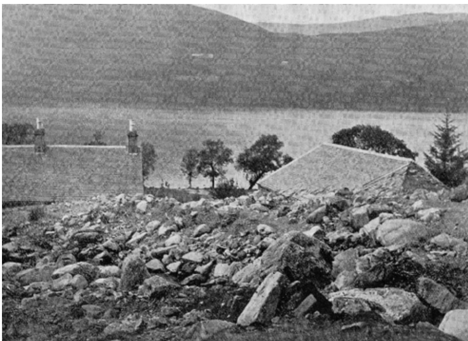
The destruction on the south side of Loch Earn
